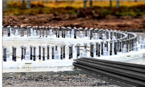
Foundation Anchor Studs
