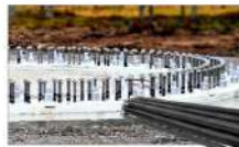
SFS: Foundation anchor studs
